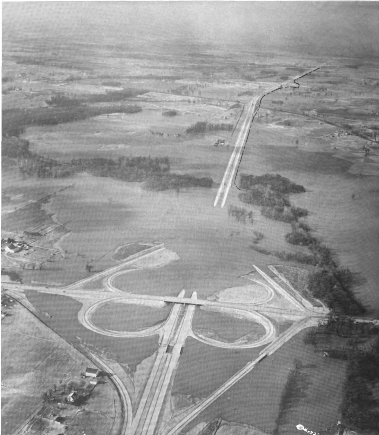
PLANNED CHANNEL WORK ALONG INTERSTATE 70. LOOKING WEST FROM THE OHIO 79 INTERSECTION, JANUARY 22, 1959.
