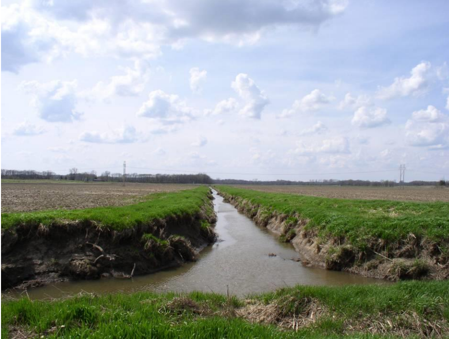
Figure 2 Looking west up a tributary of Pigeon Swamp Ditch. Bank failure caused by sapping occurs along the entire reach.
