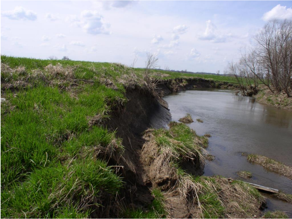
Figure5 Bank failure along the Licking River in the flood pool. Blocks breaking Away from the banks with their tops tilted toward the river. In this case the river took about 2 feet of bank or more over the length of the meander in one event.
