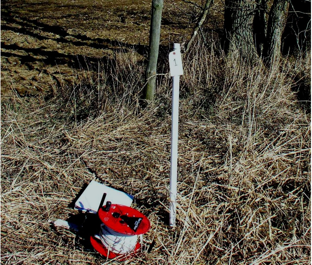
Figure A typical piezometer installation with electric water level measuring tape.
