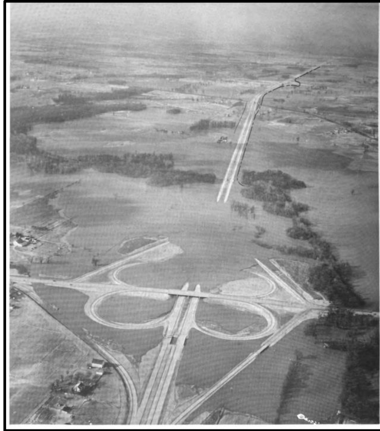
Photo: I-70 Flooding (1959); Source – SCS Original EIS and Watershed Work Plan
