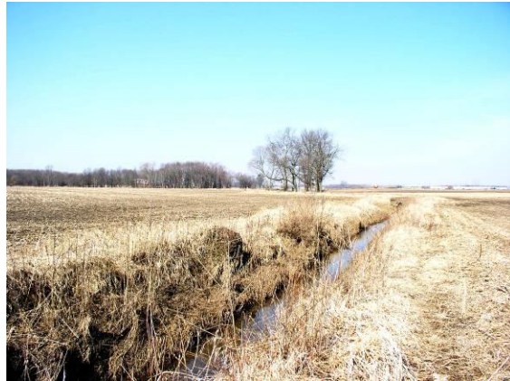
Figure 9. Stable banks along Kuhn ditch.
